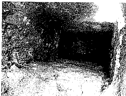
Plate 5. Brick lined chimney/flue
